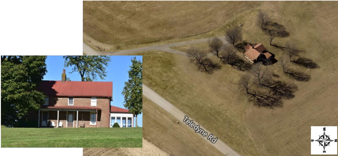
Figure 32: Potentially NRHP-eligible Resource on Teledyne Road
